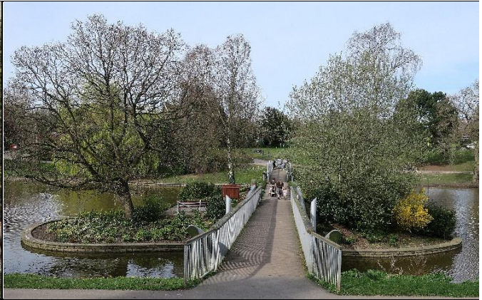
The condition of the old bridges made a replacement with a modern, stable design a necessity. The island was replanted only recently.
