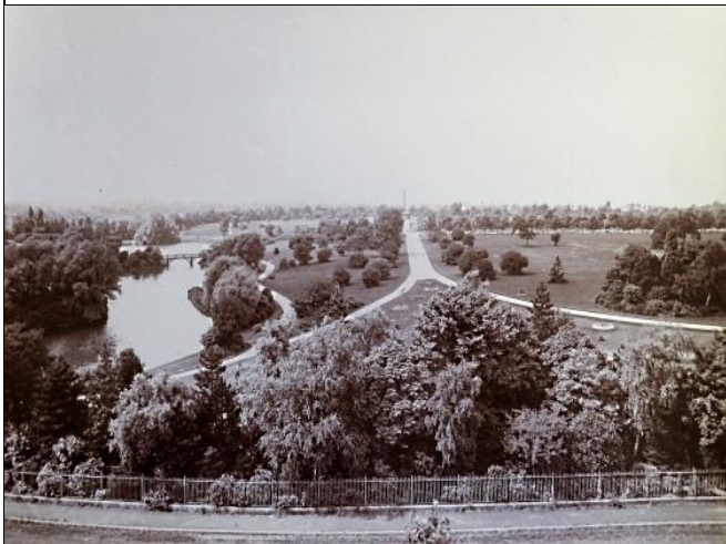
10) A 'bird's eye view' looking along the E-W axis/Broadwalk from the E. It shows the bifurcation of paths indicated in Webb's 1887 plan. Cast-iron railings separate the park from Queen's Park Drive , the circular road around the park. It is no longer possible to take this view today →
